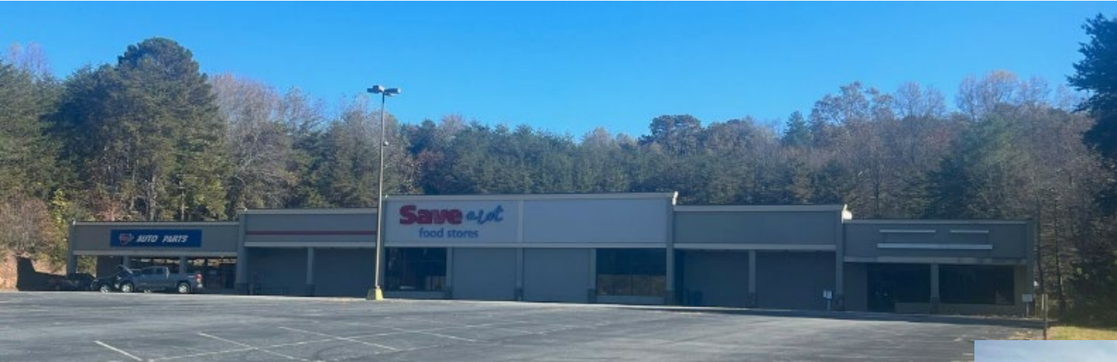
218, 226 & 238 North Main Street, Hiawassee (SAV-A-LOT Plaza)
