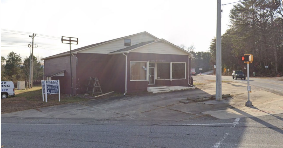
8623 Murphy Hwy, Blairsville (Abandoned Gas Station)
