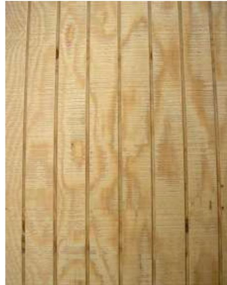
**Modern 4 foot by 8 foot T-111 exterior siding panels is inappropriate for exterior repairs or additions.**
