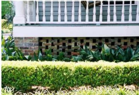
**The use of wood or brick lattice design is more desirable than using solid materials for foundation infill to provide proper ventilation and to preserve the historic character of the building.**
