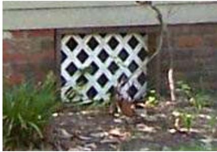
**A recommended foundation treatment for pier infill on houses originally without underpinning is to recess the new infill walls back with a short retaining wall near ground level, paint the set-back infill wall black, and install wood lattice in front of the recessed infill wall. The appearance of an open foundation on brick piers can be achieved and contemporary climate control is accommodated.**
