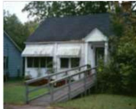
**Example of inappropriate placement and lack of screening of handicap access ramp.**
